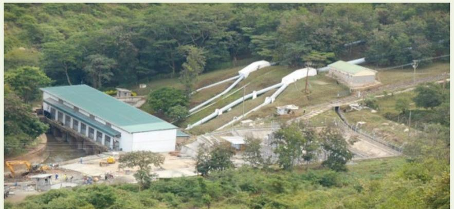
*The photo shows the rehabbed Wanjii powerhouse, penstocks, winch track and trolley. The evacuation substation was done anew to improve the substation performance. The Winch allows ease of access for staff and equipment to the powerhouse. A road was constructed to the powerhouse to improve access.*
